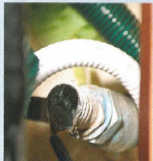
The cracked toilet outlet tailpipe left an irregular hole to block
